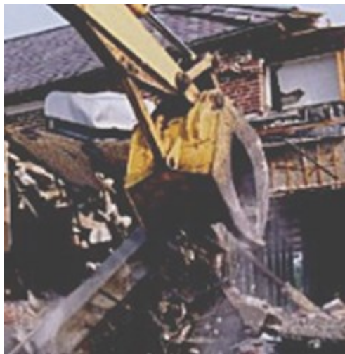
▲ High-speed demolition by machine is the norm.
