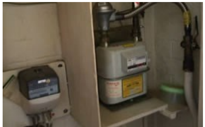
▲ An asbestos panel used around a gas meter.
