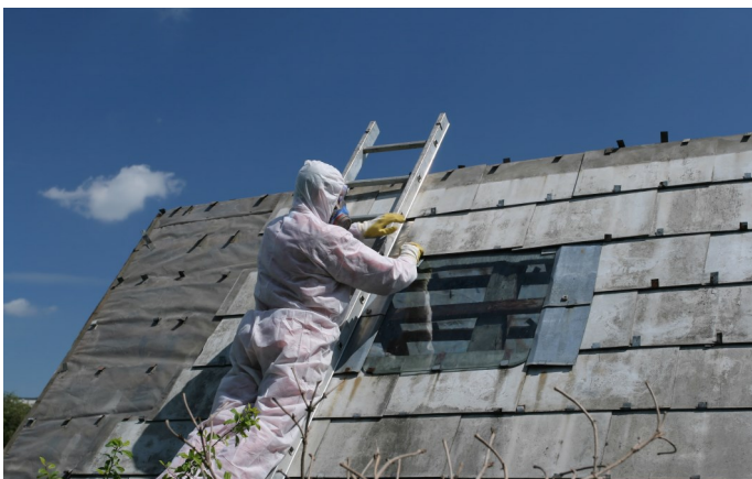
▲ Asbestos roof tiles, typically used on industrial and agricultural buildings.
